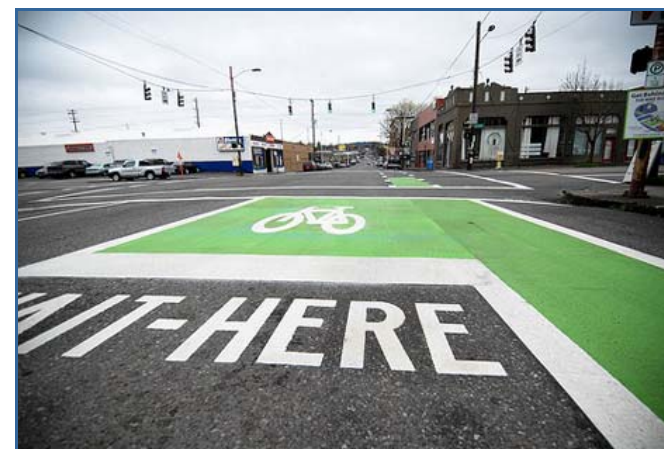
Figure 21: Photo of Bike Box Installation
