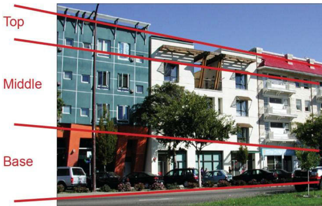
Figure 4.6.2.g: Photo example of buildings that satisfy the massing and articulation standard for a base and top that are human-scaled.
