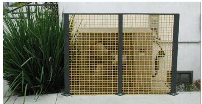
Figure 4.7.3.d: Photo example of an exterior utility screen designed to complement the architectural design of the building.
