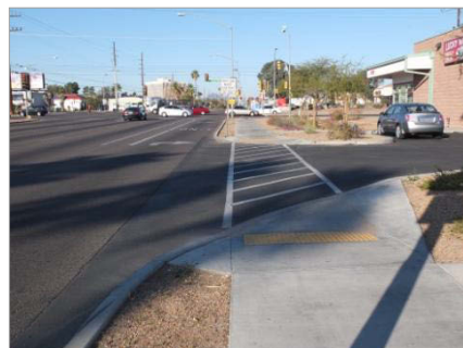
Figures 4.4.4.v and 4.4.4.w: Diagram and example photo of a dropped driveway condition that does not satisfy the GRD standards.
