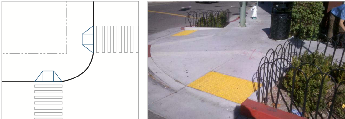
Figures 4.4.4.r and 4.4.4.s: Diagram and photo example of directional curb ramps.
