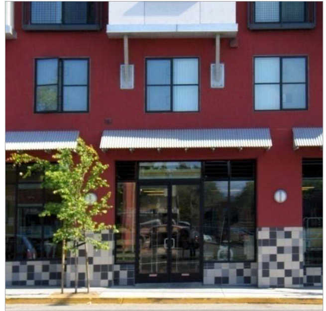
Figure 4.6.2.r: Photo example of a main entrance that has composition and articulation that make it human-scaled.
