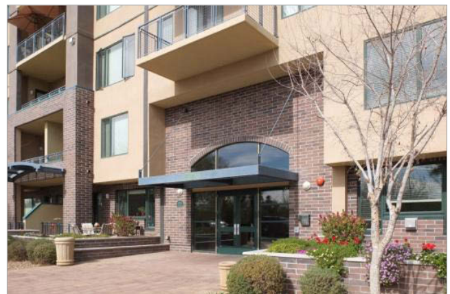
Figure 4.6.2.s: Photo example of a clearly defined building entrance. This lobby entry is distinguished from the individual unit entry to the left by its large-scale awning and the entry plaza.
