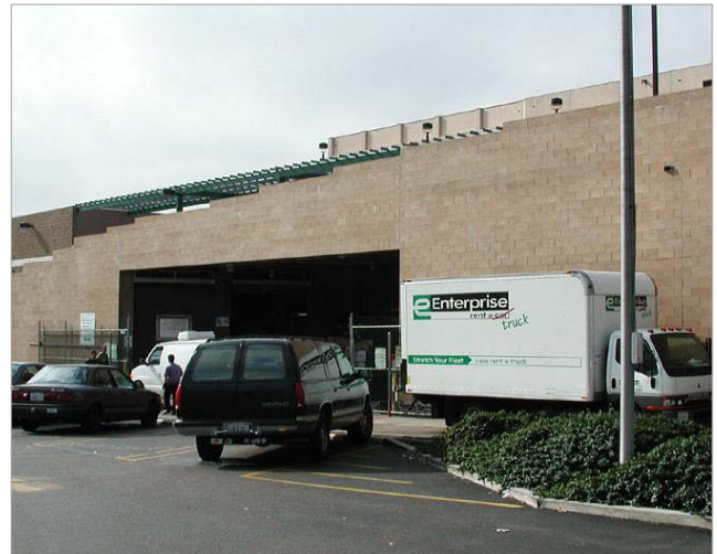
Figure 4.7.3.a: Photo example of loading facilities within the building envelope.
